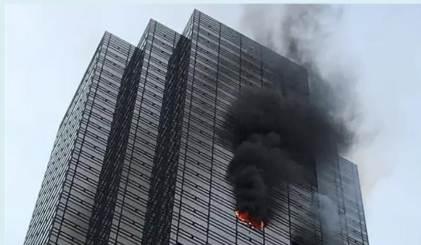
Fire damage in New York (USA)
